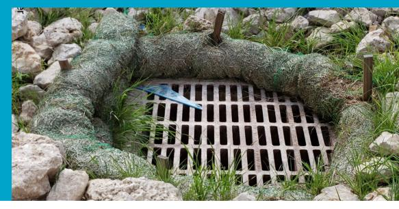
ditches, gutters, storm drain, and other engineered collection systems and is discharged ultimately into the Inner Harbor. The stormwater runoff often carries trash, hydrocarbons, heavy metals, and other pollutants.
