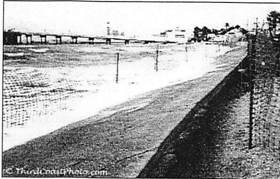
After erosion caused the Beachwalk to collapse, the city secured emergency funding to repair it.
